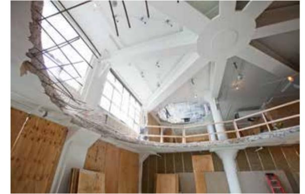
It took three months to install the asterisk-shaped steel structure that stabilizes the opening for the Coin Stair.
