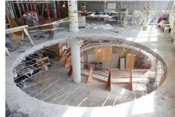
One column was removed to accommodate the lower staircase: the Coin Stair. Thanks to a structure added for reinforcement, the four floors above can support the approximately 975 kg per m<sup>2</sup> for which the building was originally designed.
