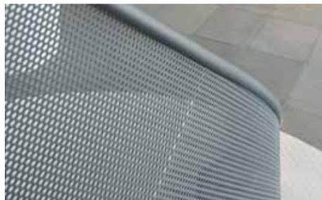
**PERFORATED METAL SHEETS** were made by Brakewell and assembled by SNC Contractors.
